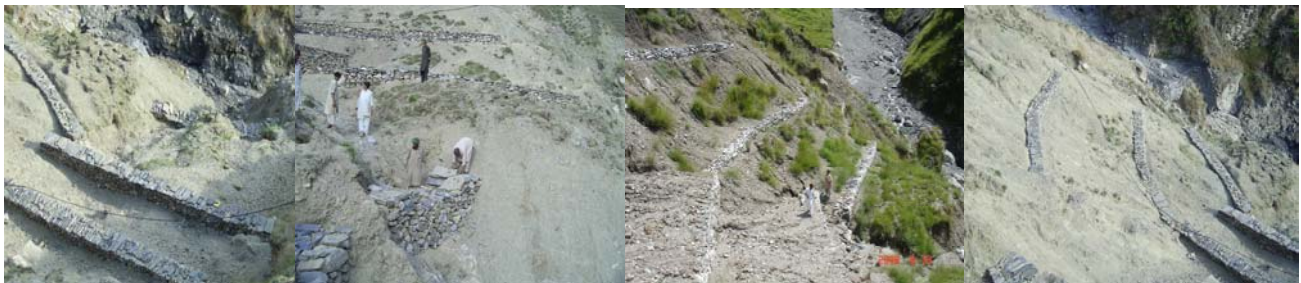
Check dam construction in Gulmera Batora Watershed in NWFP 2008
