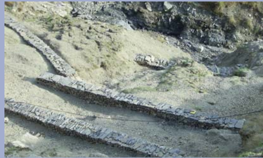
Stone bunding for soil conservation at Gulmera Batora watershed
