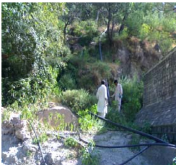
Pipes installed for irrigation water, Dhani Mai Sahiba village, Muzaffarabad PAK
