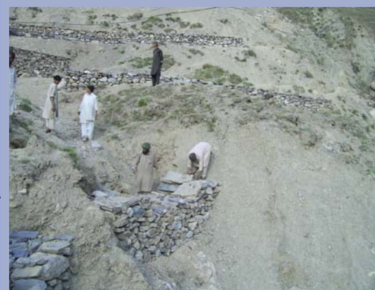
Check dam repair in Gulmera Batora watershed
