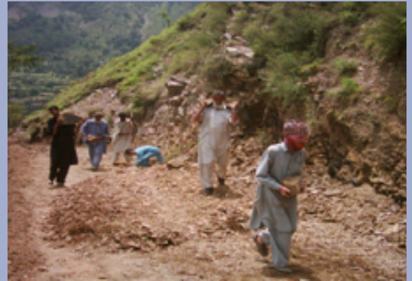
Widening of village link-road at Pekho Nakar Union Council Abbottabad district (NWFP) in the context of the Livelihoods Rehabilitation Strategy of ERRA supported by FAO.
